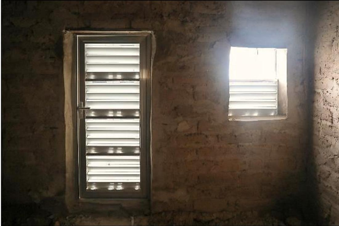
Figure 4. Photo of interior of a home in Wellingara Village, The Gambia, after installation of mosquito exclusion doors and windows. The doors feature perforations for ventilation, and transparent panels to allow light to enter the home, as shown. Perforations in the doors and windows are too small for mosquitos to pass through. *Photo: Steve Lindsay (Durham University).*
