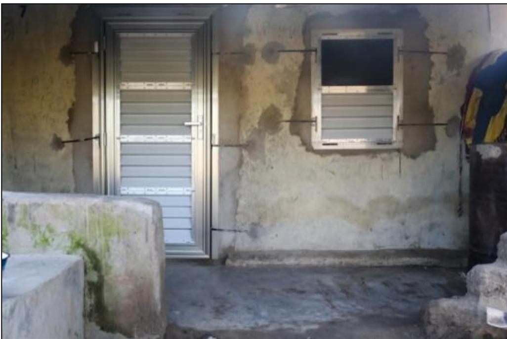
Figure 3. Photos of an entry way to a home in Wellingara Village, The Gambia, before (top) and after (bottom) installation of mosquito exclusion doors and windows. The home is one of thirty (30) houses participating in a pilot field evaluation of the doors and windows. The field evaluation began with door installation in August 2017. *Photos: Steve Lindsay (Durham University).*
